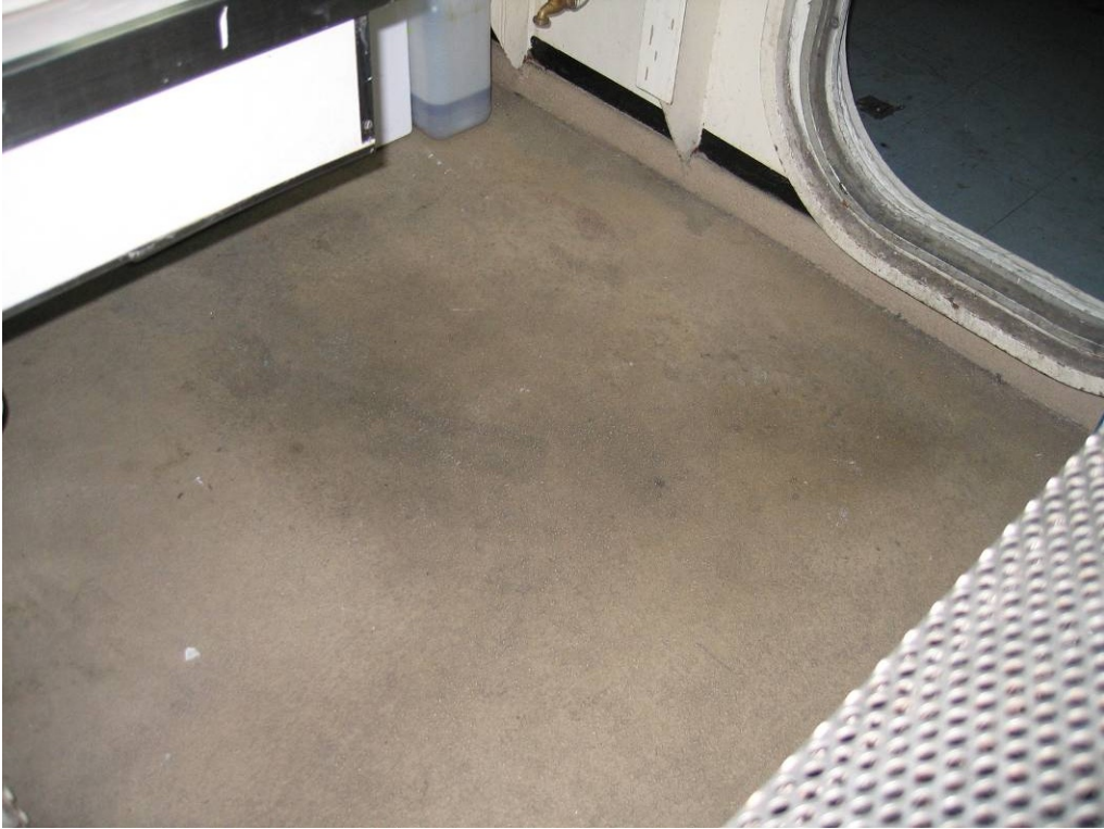
The deck surface just inside the access.
