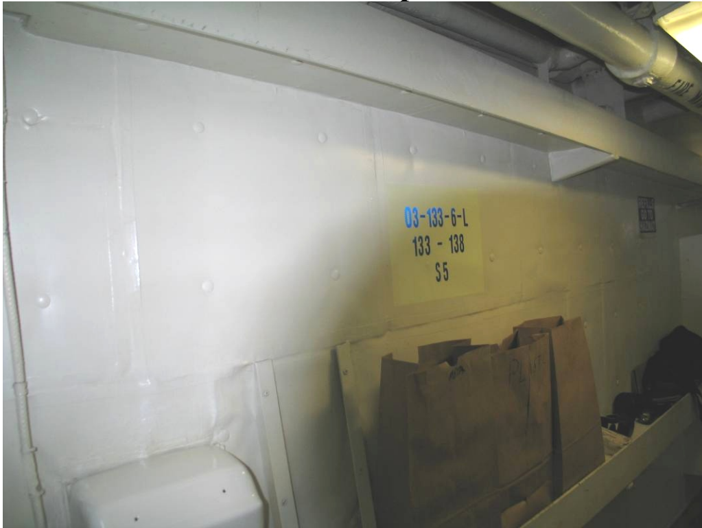
Space identification placard (“bullet”). This washroom has exposed framing, piping, etc.
