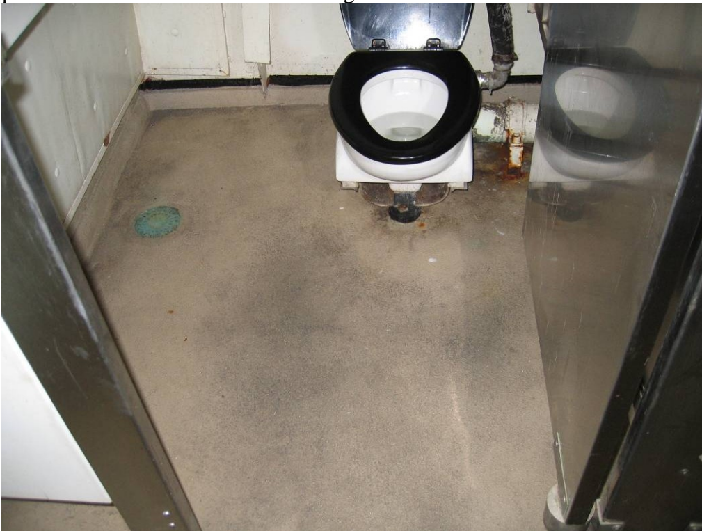
All rust stain observed is running down from appendages or is metallic fragments corroding on the surface of the coating. The deck coating is in excellent condition.
